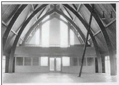
Inside looking towards Water Street
